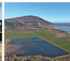
Replacing aging water control structure at Petite-Ferme to preserve ecological integrity. PHOTO CREDIT: DU CANADA
