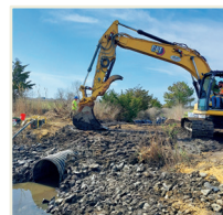
Replacing aging water control structure at Manahawkin WMA, NJ that will be resilient to climate change and sea level rise. PHOTO CREDIT: NJDEP
