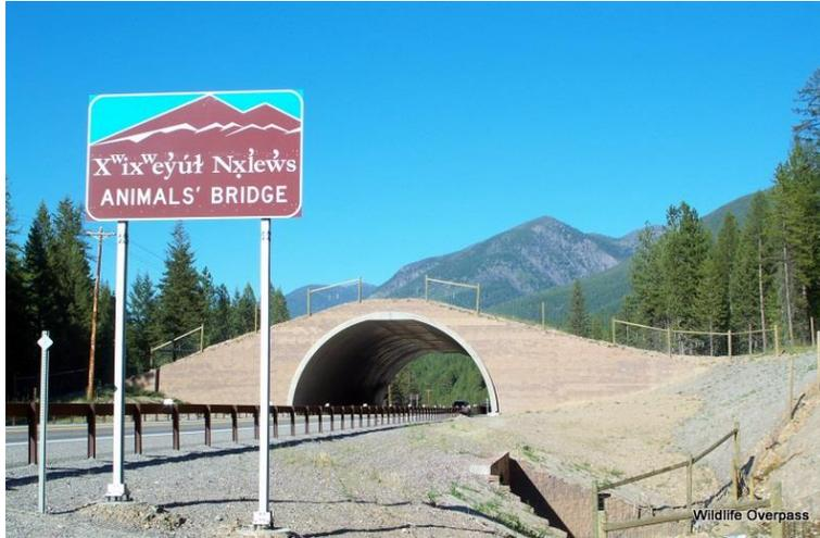
Figure 14. A wildlife overpass constructed on US Highway 93 in Montana. (Confederated Salish and Kootenai Tribes)
