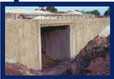
Culvert, Photo Courtesy of USGS
