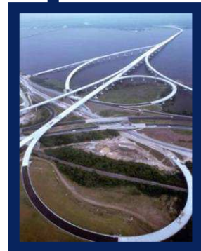
Neuse River Bridge, Photo Courtesy of DOT
