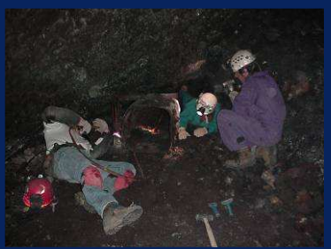
Installing a Cave Gate, Photo Courtesy of NPS
